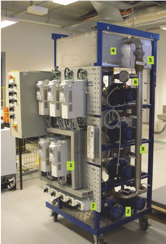
Fig. 6. Experimental setup: (1) ACQ810 frequency converter; (2) EbaraCDX120/12 centrifugal pump; (3) pipeline with 2-inch inner diameter; (4) fluid reservoir; (5) throttling valve; (6) pressure sensor.
