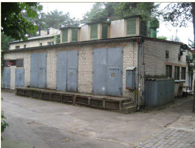
Fig. 1. 10 th substation of electrical network in city Riga.
